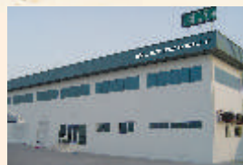
PLANT II, DUBAI
