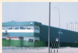
PLANT I, DUBAI
